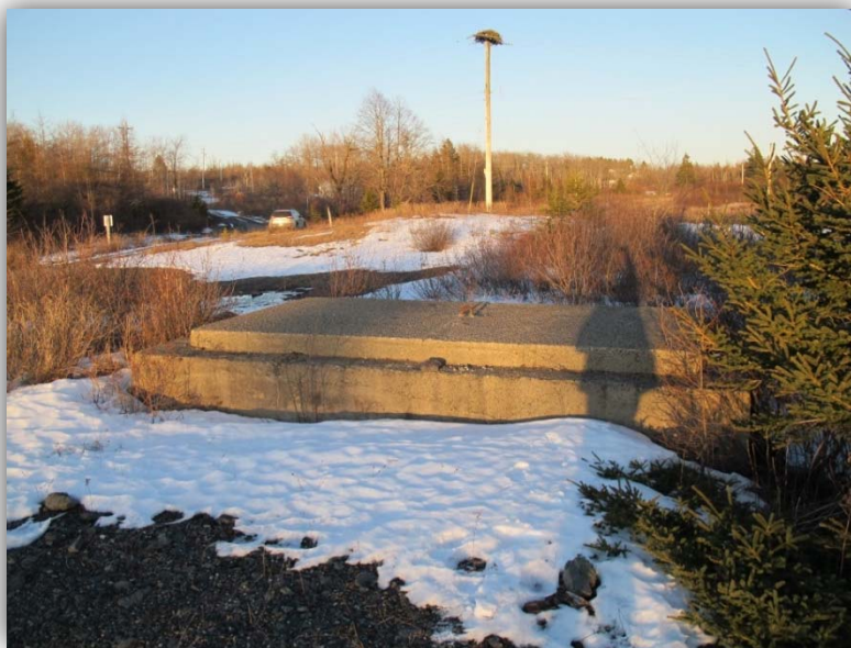
Figure 22 - Stuart Shaft capped by a 1990s cement cap.
